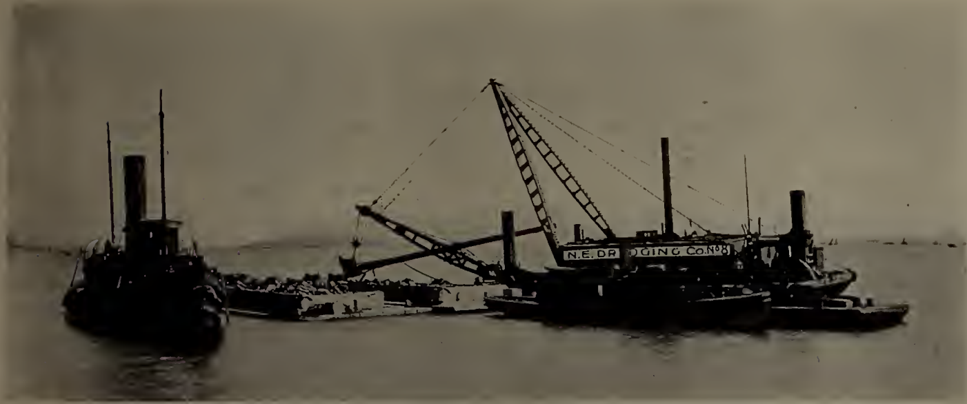
NEW ENGLAND DREDGING COMPANY'S SCOOP DREDGE NO. 8 IN OPERATION. Office, 12 Post Office Square, Boston.
